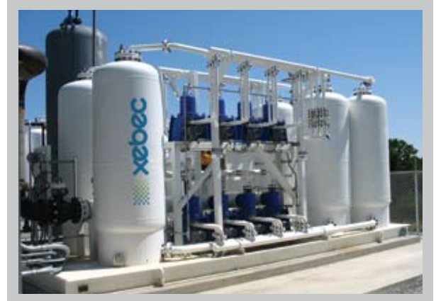
The XEBEC M-3100 gas purification system at Rumpke landfill provides pipeline-grade natural gas to Duke Energy customers in Ohio.
